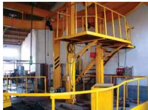
TEST PLATFORM FOR HOIST UP 7.5T
